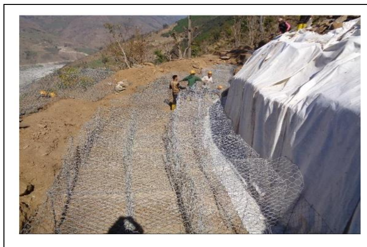
Figure 7-2: Laying Geotextile filters and Gabions before filling stones
