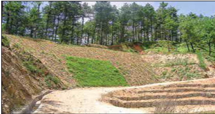
Figure 8-6: Sod Facing (Turfing)
