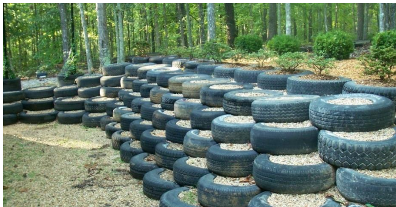
Figure 7-11 Rubber Tires filled up and used for river protection
