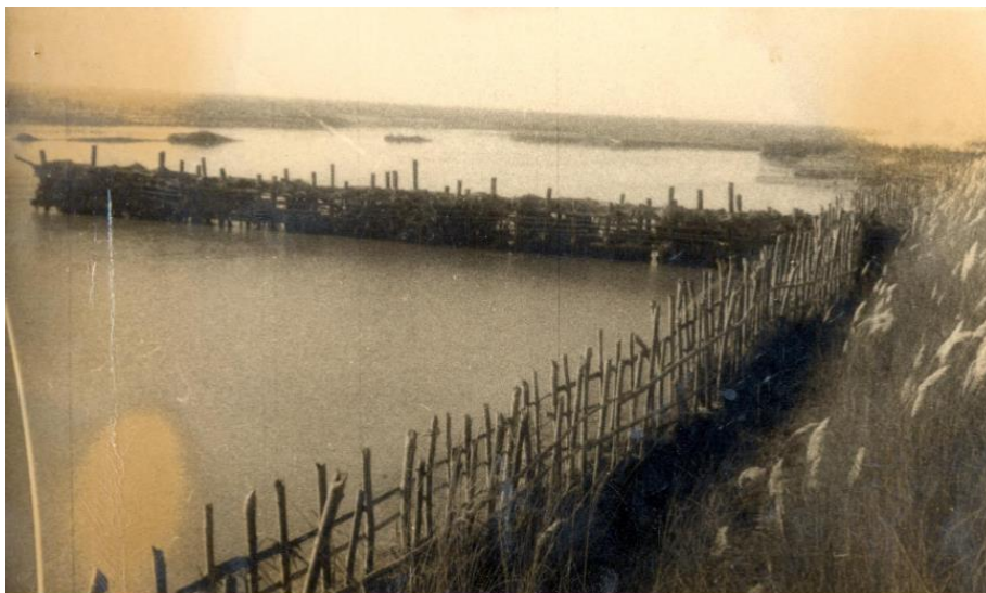
Figure 7-12 Bamboo screen and Permeable Spur
