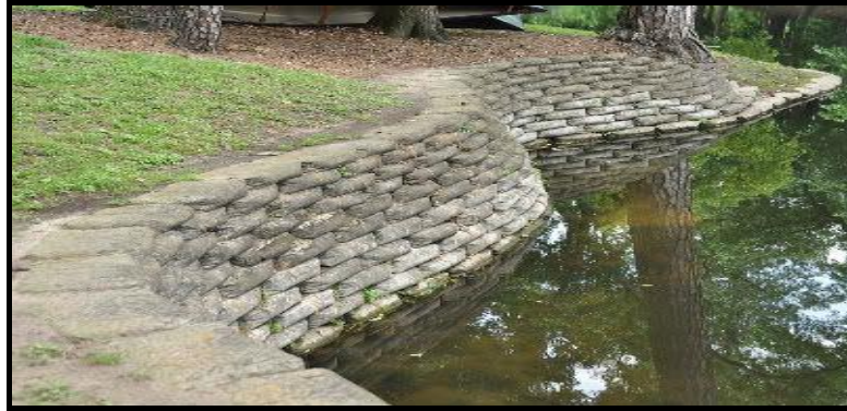
Figure 7-10 Sand Bags Wall Used for River Training Works
