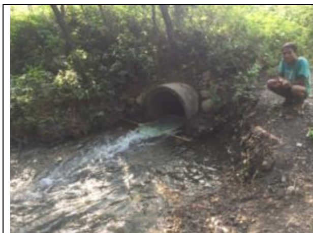
Piped irrigation inlet in Girwari Khola embankment
