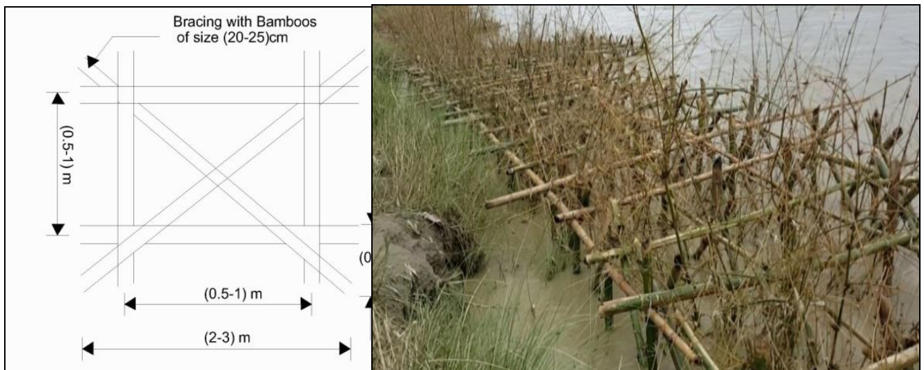
Figure 7-7: Bamboo Porcupine as Damper for Bank Protection
