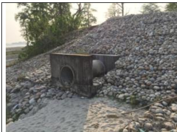
Ungated outlet in Karnali embankment near Jagatpur, Kailali
