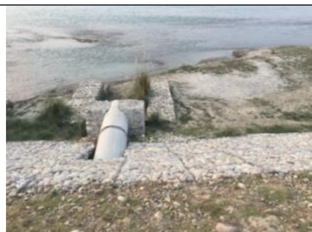
Drain outlet in Karnali embankment near Anantapur, Bardiya
