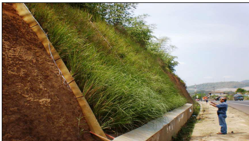
Figure: 8-7 : Vetiver for Slope Stabilization (Slope > 80°)
