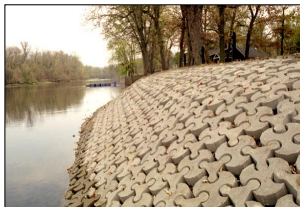
Figure 7-3: Concrete Dolos and Interlocking Blocks as Revetment
