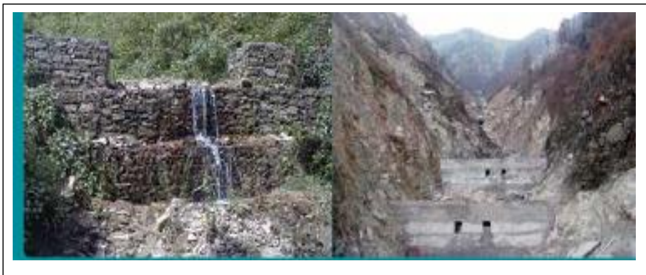
Figure 6-17: Check Dam to control erosion and Gully Plugging (Source ICIMOD Resource Manual)
