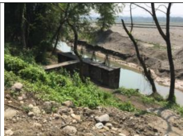
Gated irrigation intake at East rapti dyke
