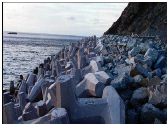
Figure 7-3: Concrete Dolos and Interlocking Blocks as Revetment
