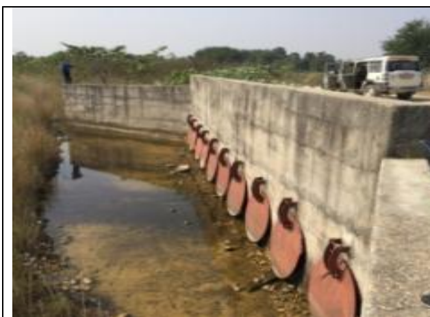
Anti-flood sluice in Kamala embankment near Sagara, Dhanusha
