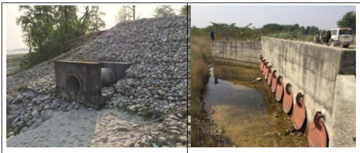
Figure 6-6: Images of typical flood sluices (ungated ) in Karnali embankment and gated flap valve in Kamala Embankment.
